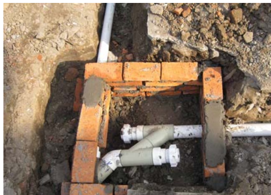
check well in construction
