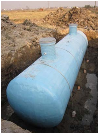
black water box in installing
