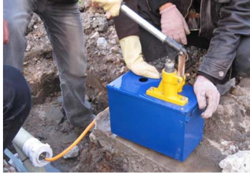
pressure test of the vacuum pipe-line
