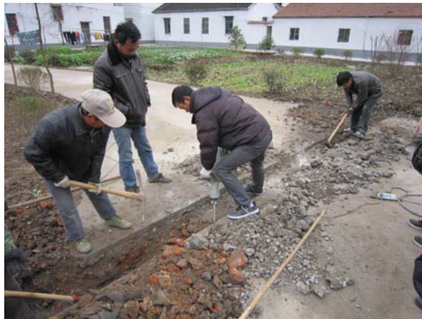
excavation for vacuum pipe-line
