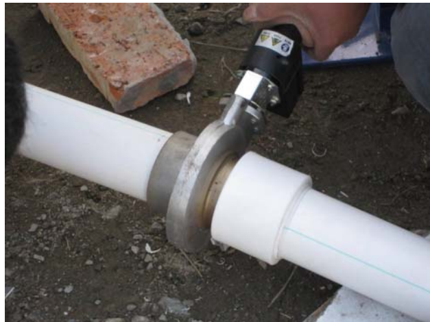
butt fusion welding of the vacuum pipe-line
