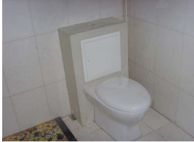
installed vacuum toilet
